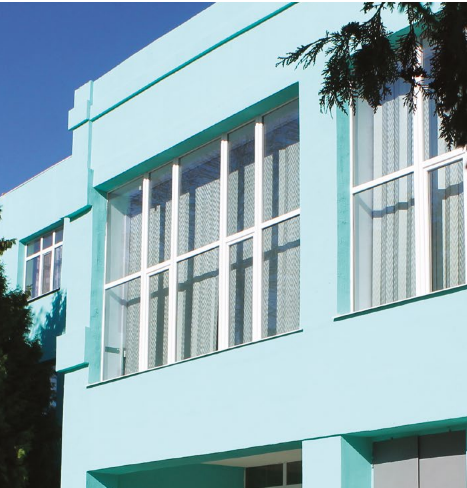
Nova Galeschina school refurbishment, September 2020.
