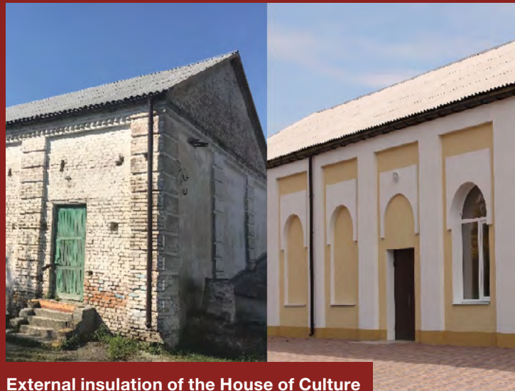
External insulation of the House of Culture in Novogaleshchinskaya ATC
